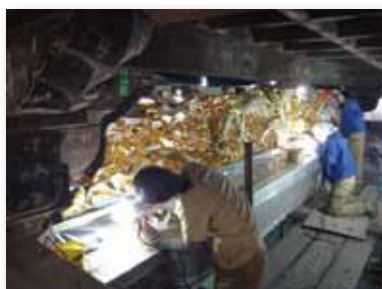
Repair work on the Kara-mon Gate
