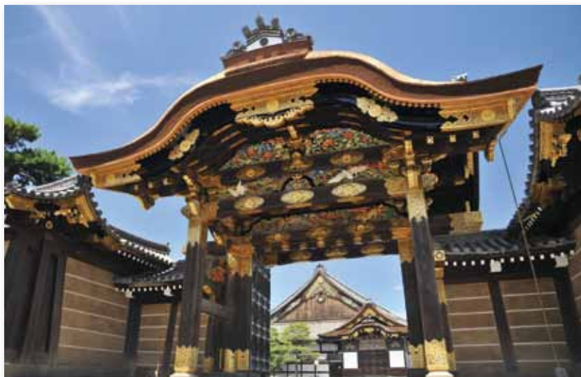
Kara-mon Gate: repaired in 2013
