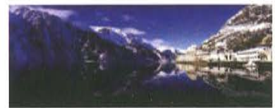
Tyssedal Hydropower Station, 1908, at the head of the Hardanger Fjord in Odda, Norway
