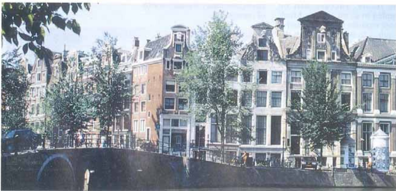
Late 17th century canal houses along Herengracht canal
