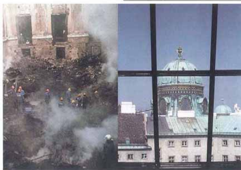
LEFT : The cleaning-up operations at the Large Assembly Hall immediately after the fire of November 26-27, 1998.
