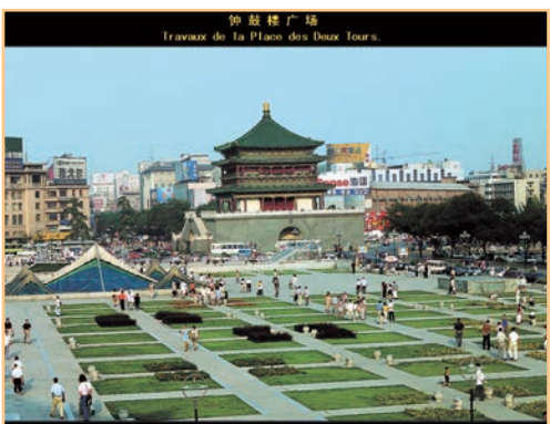
[Xian-1] The Bell and the Drum Towers Square Construction Project: The Bell and the Drum Towers Square is a comprehensive project involving both preservation of relics and renovation of Ming city. The whole project is integrated with underground space exploration, city-greening, relics preservation, and development of commercial facilities.
