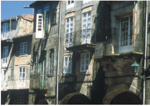
The people identify the protection of cultural heritage with the restoration of the natural environment.
