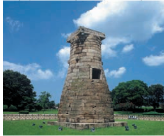
Cheomseongdae Observatory is a scientific structure and every stone used in its construction has its own symbolic meaning.
