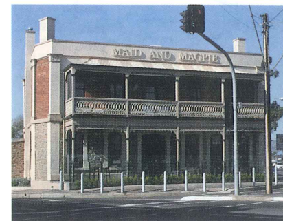
...and after refurbishment was completed in 2007.
