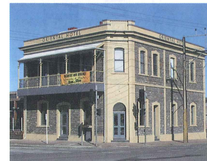
...and after refurbishment was completed in 2008.
