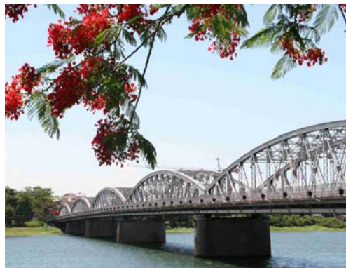
Trang Tien Bridge - Huong River
