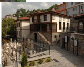
(Photo 8) Seyyid Usul Lodge after the restoration (Seyyid Usul Lodge Culture Center)
