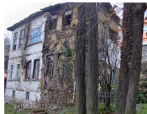
(Photo 7) Seyyid Usul Lodge before the restoration
