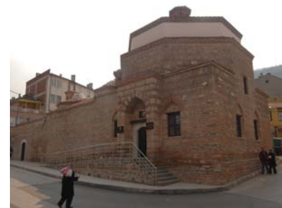
(Photo 4) Turkish Bath of Murat II. after the restoration (Turkish Bath of Muradiye Center for Handicapped)
