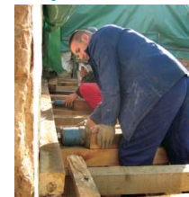
Correction of the northern wall with hydraulic presses
