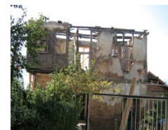
Panjina Tower - dismantling of the building, 2009
