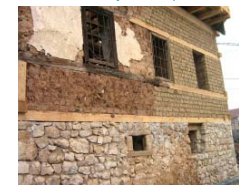
Combination of the existing and new clay-brick in the southern wall
