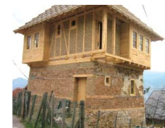
Wood, clay-brick and stone - traditional materials applied during the works
