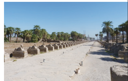
Restoration of the Avenue of the Sphinxes
