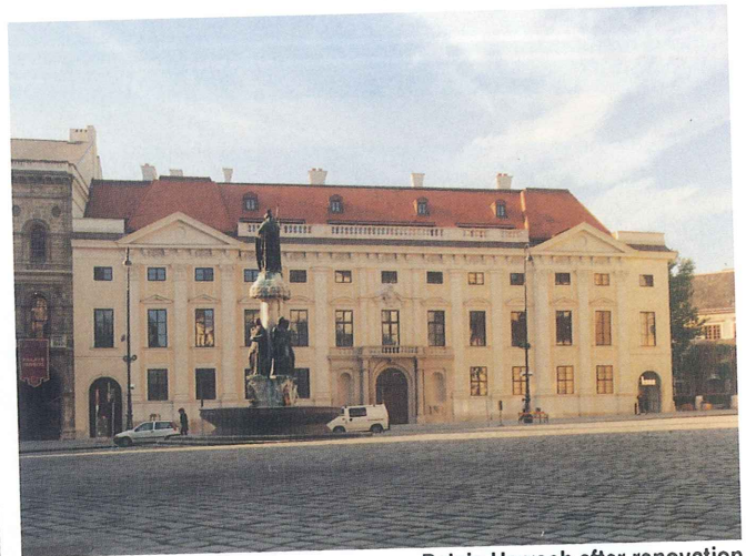
Palais Harrach after renovation
